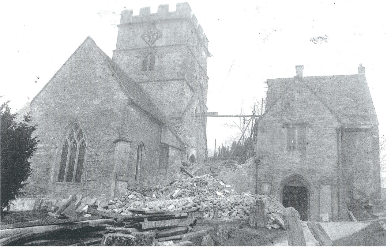
After the wall collapsed, 10 December 1902
