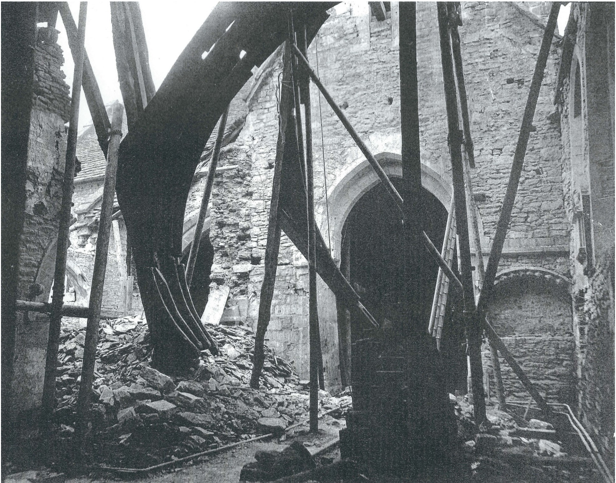
Inside the church after the wall collapsed, 10 December 1902
