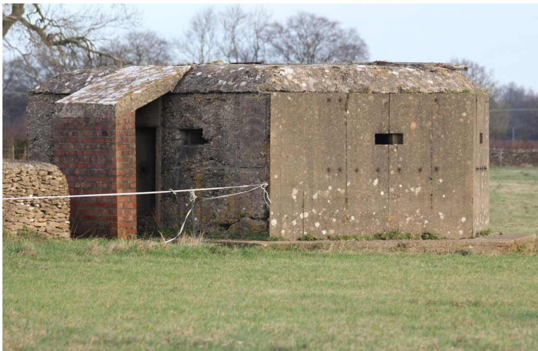
Figure 400 - Feature 4. Pill Box Type 24 Photo taken from the south west.
