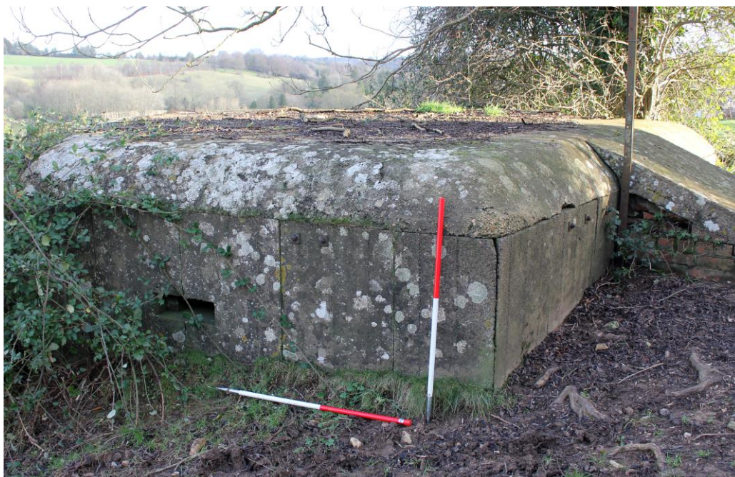
Figure 200 – Feature 2, Pill Box Type 24. Photo taken from the south looking north.
