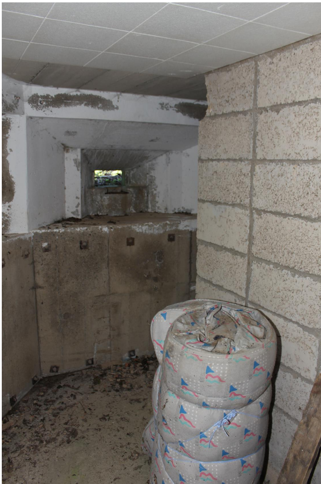
Figure 602 – photo indicating modern additions including a mattress, paint on the walls and polystyrene roof panels
