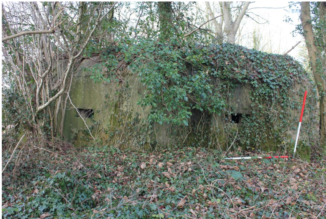
Figure 700 – Feature 7 – Pill Box Type 24. Photo taken from the south looking north
