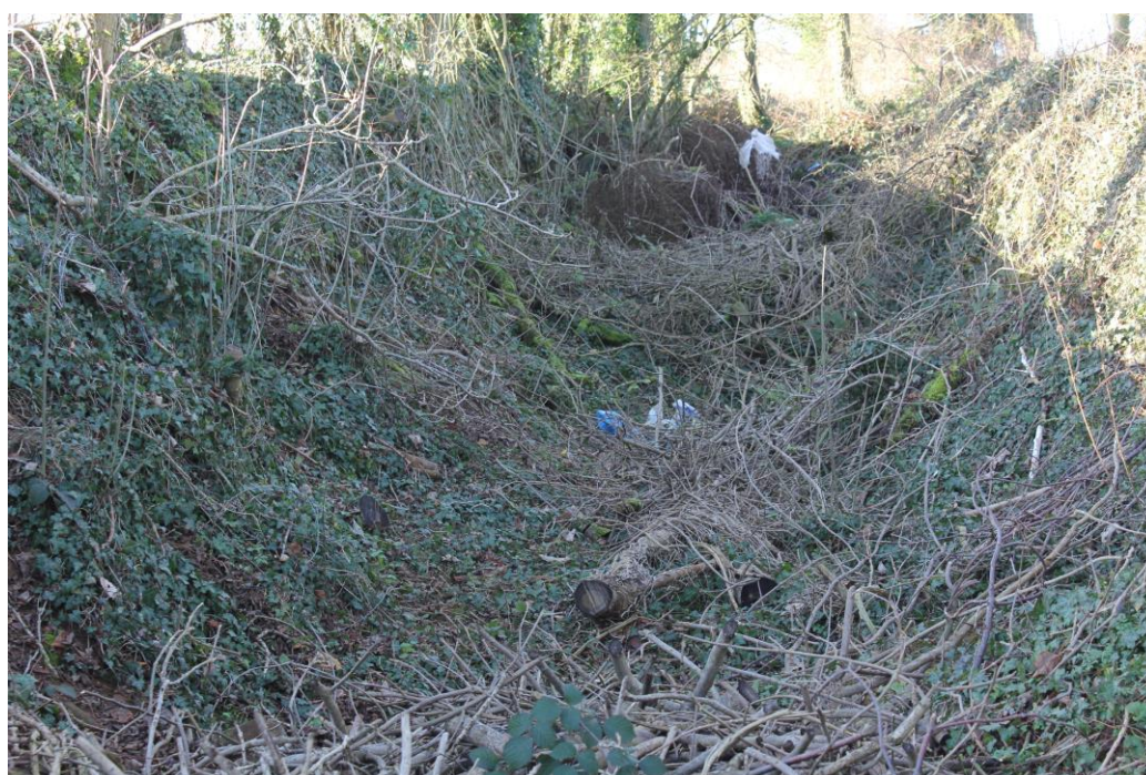
Figure 501 – photo indicating the build up of rubbish in the anti-tank ditch, feature 5
