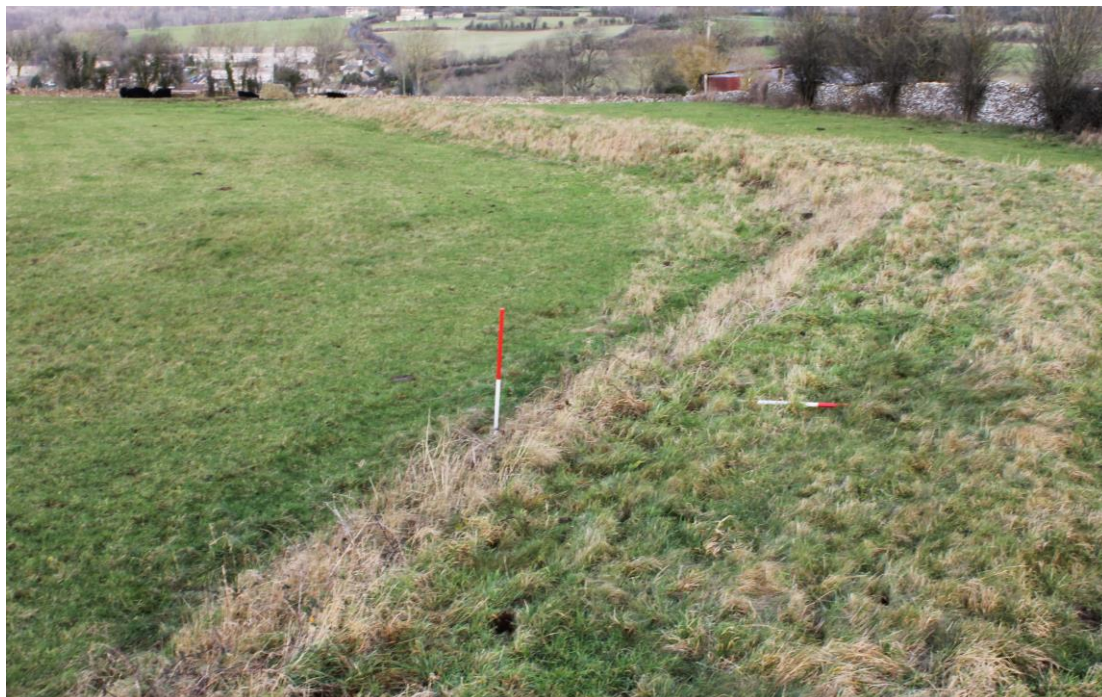
Figure 302 – Looking towards feature 2 down the anti-tank ditch towards the end of part 1 on drawing 300
