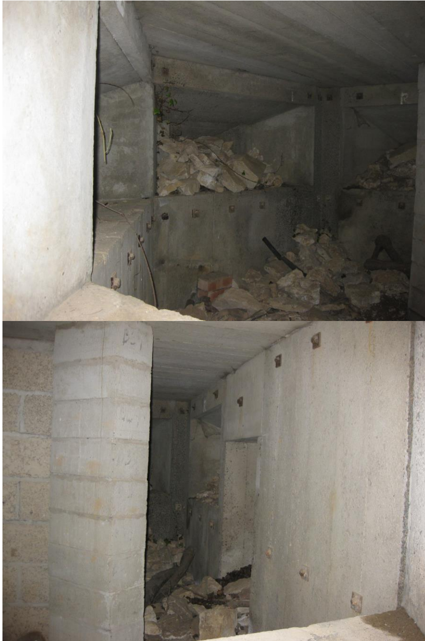
Figure 203 – Rubble starting to build up in the pill box.
