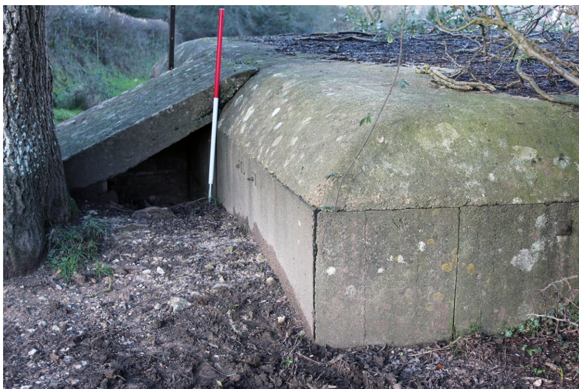
Figure 202 – Entry porch to the pill box, semi-sunken by soil
