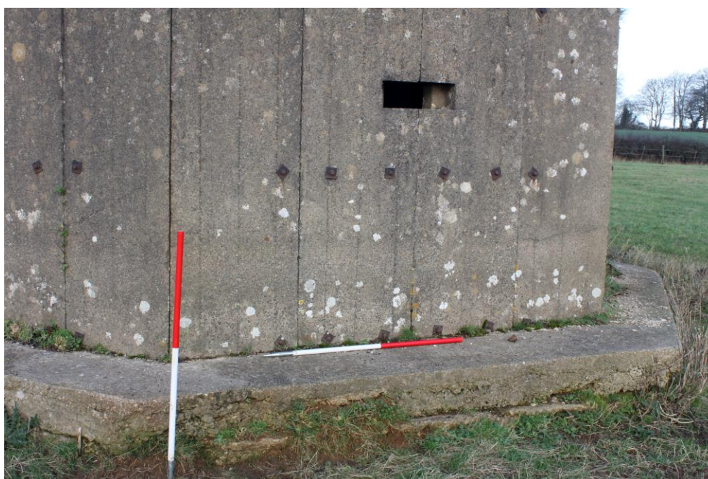
Figure 401 – internal (top) and external prefabricated concrete panels and iron bolts on feature 4
