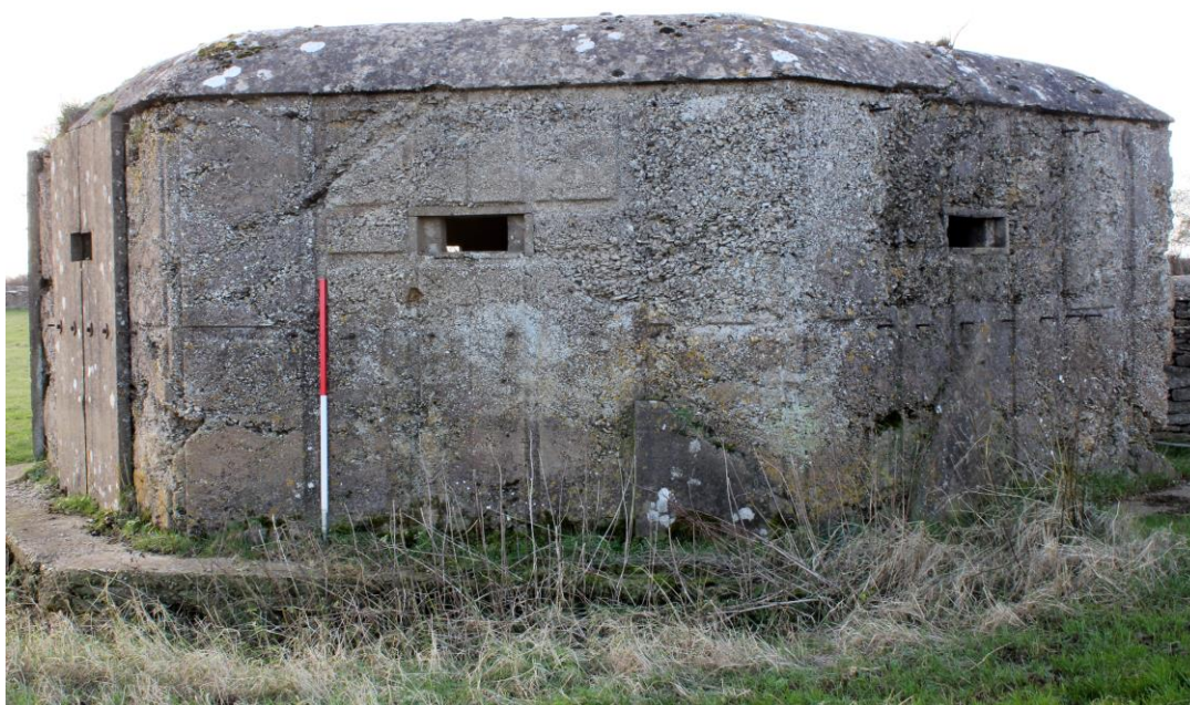
Figure 403 – photo indicating the damage to the outside of feature 4 which is not visible from Star Lane (photo taken looking towards the lane)
