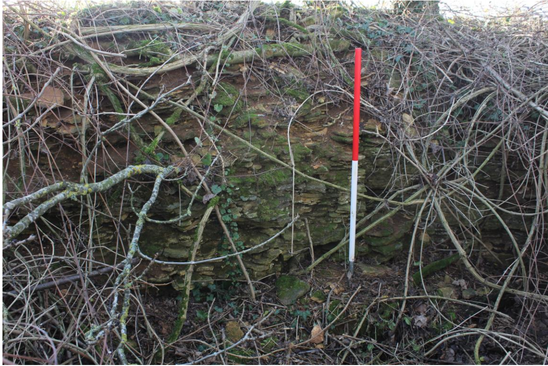
Figure 502 – photo indicating the wall of the anti-tank ditch
