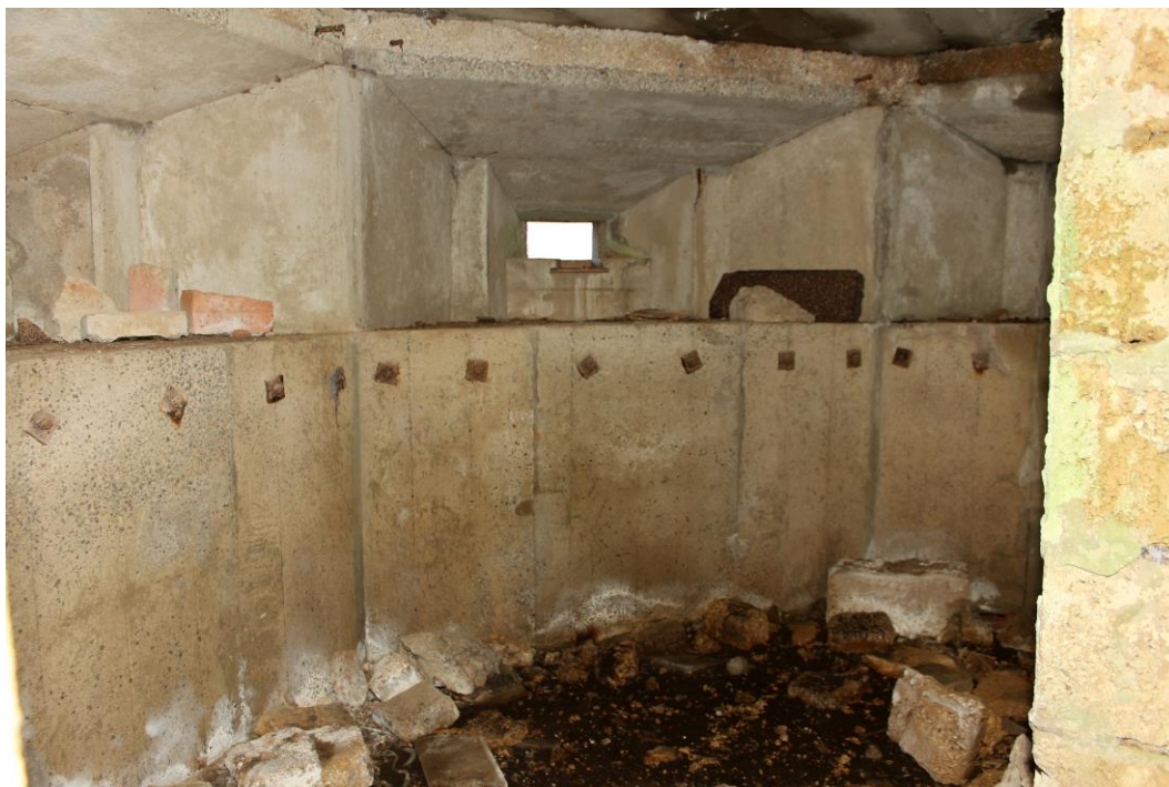
Figure 401 – internal (top) and external prefabricated concrete panels and iron bolts on feature 4
