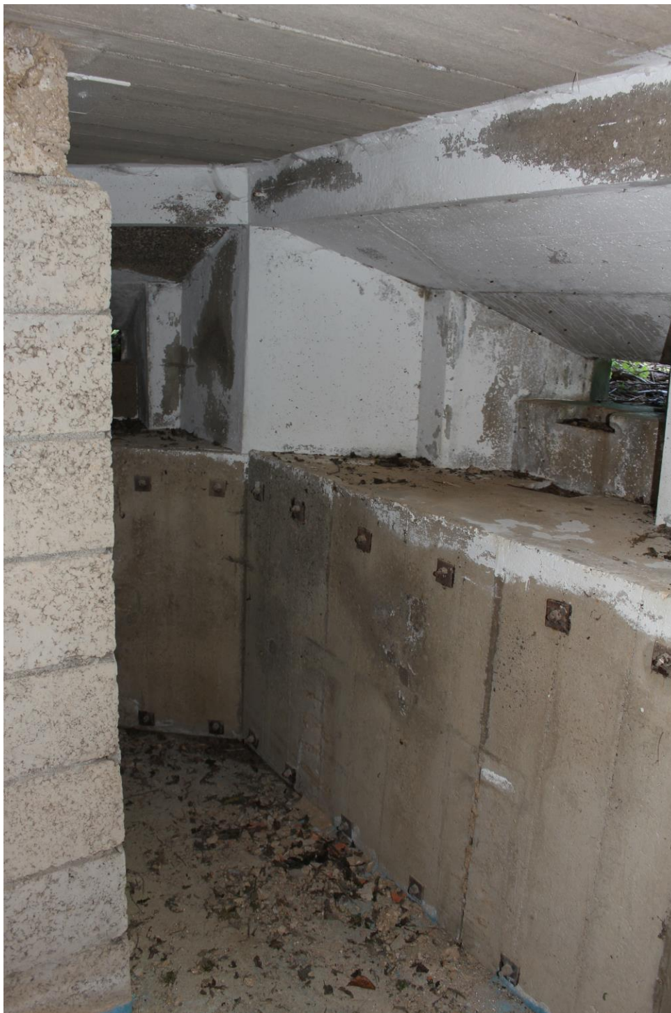
Figure 601 – interior prefabricated concrete panels and iron bolts.
