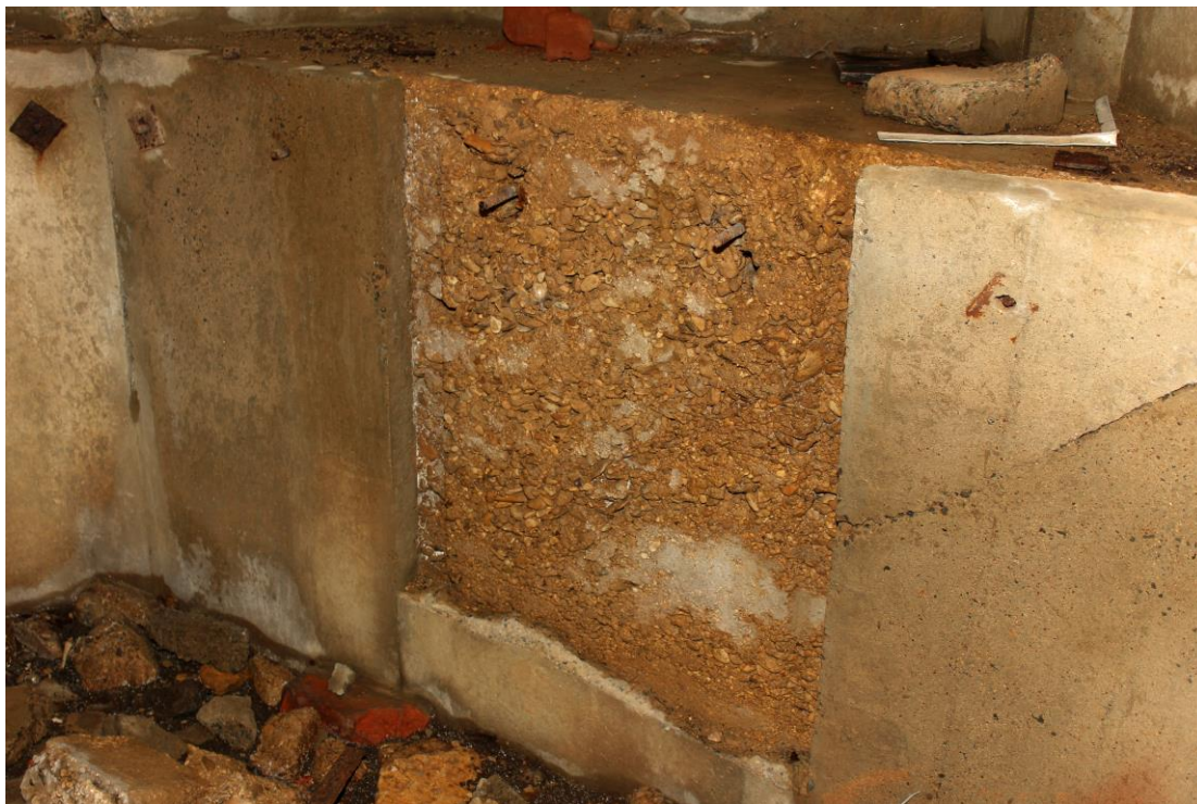
Figure 402 – photo showing some of the damage what has occurred to feature 4.
