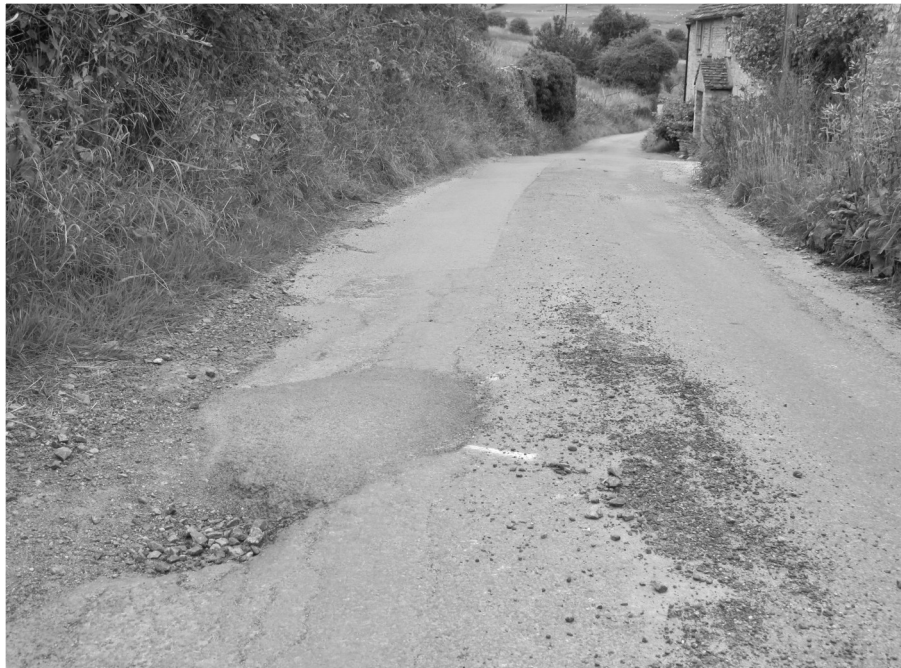
Potholes on Westend - soon to be a thing of the past?
