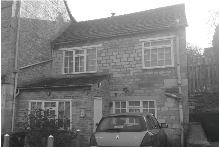
The old post office at the bottom of Point Road
